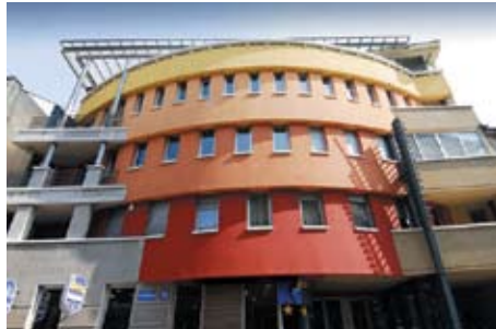
■ Stambeno - poslovni objekat, Beograd Residential - Office building, Belgrade
