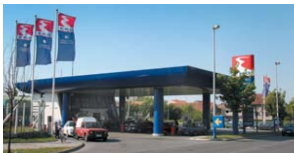
■ Benzinska pumpa MALEX OIL, Novi Beograd Gas station MALEX OIL, New Belgrade
